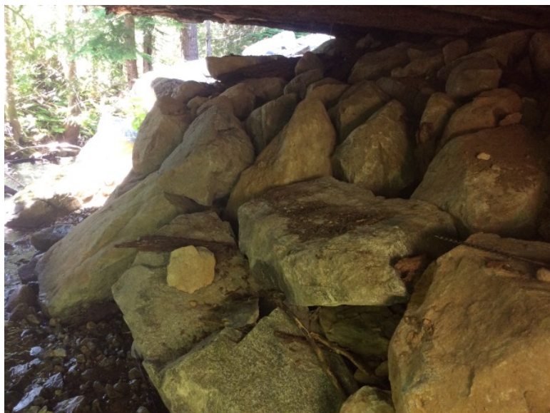
Right Bank Abutment when facing downstream
