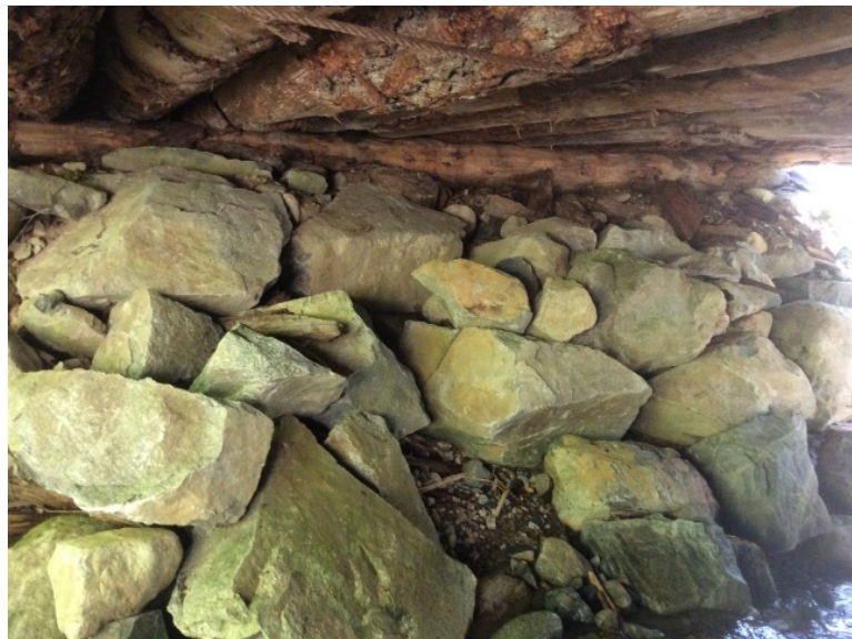
Left Bank Abutment when facing downstream
